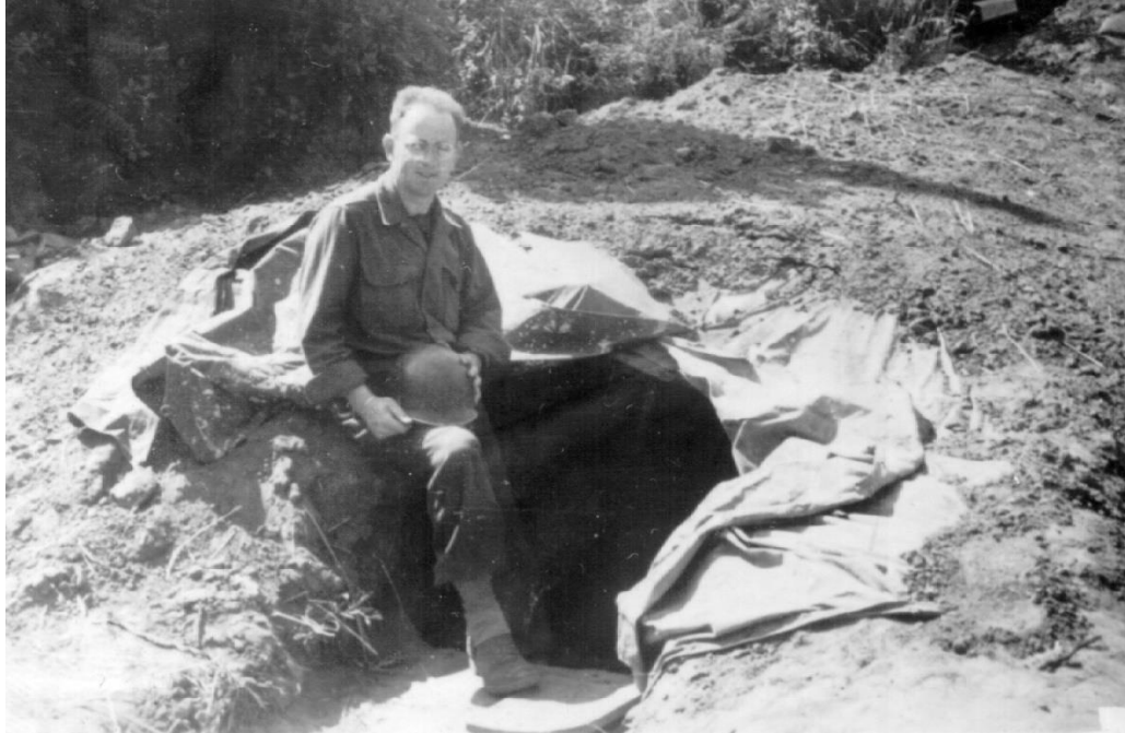
REF at tunnel entrance
