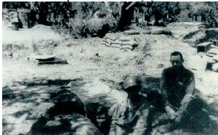
Tunnel Entrance at Anzio
